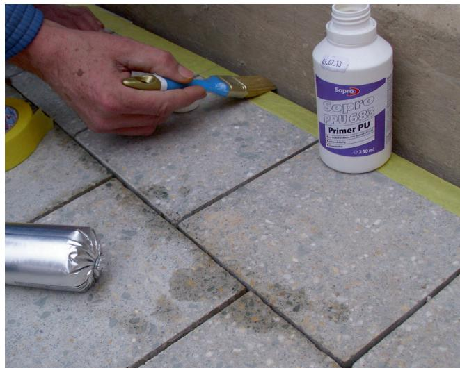
1 Mask joint with adhesive tape and pretreat with Sopro PPU 683 PU primer.
