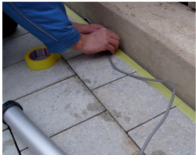
2 When Sopro PPU 683 has dried, insert circular-section PE back-up strip.
